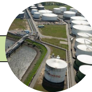
Ammoniak-Terminals in Hamburg/Brunsbüttel
